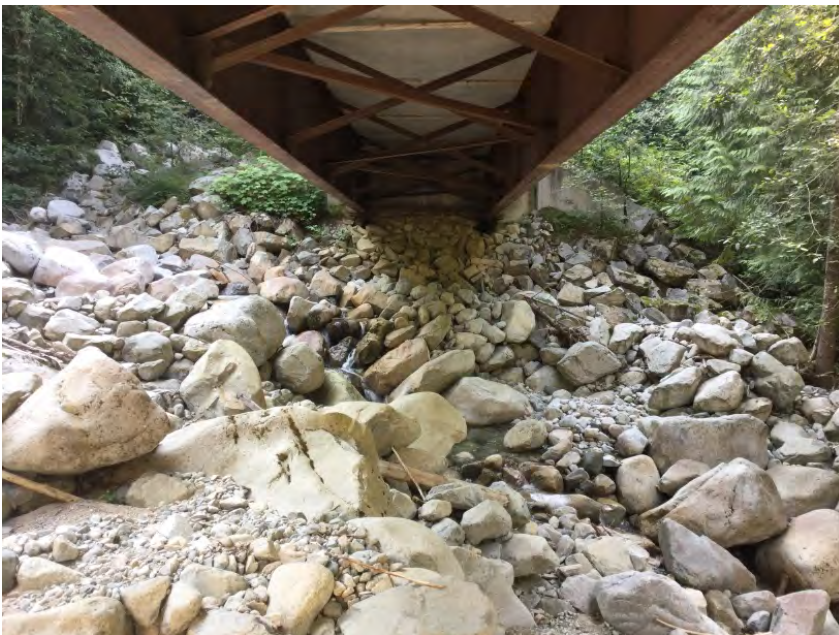
Left Bank Abutment when facing downstream
