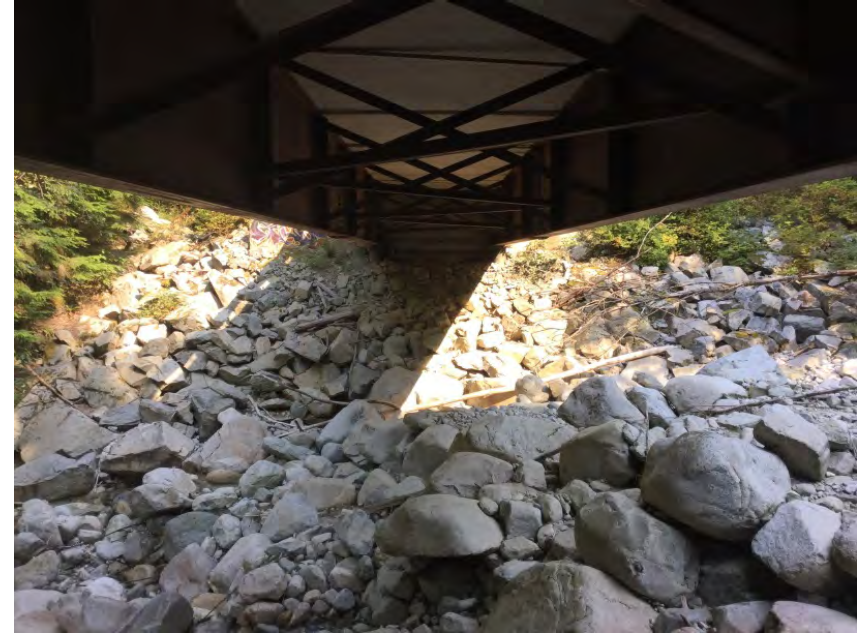
Right Bank Abutment when facing downstream
